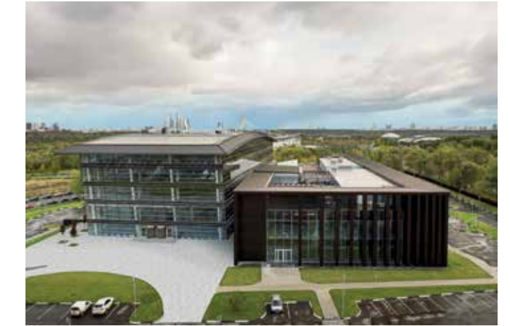
Commissioning of B5
