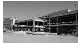
Commissioning of the B1
